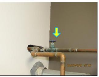
6.2 Item 5(Picture) corrosion near water heater
