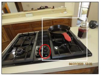
11.5 Item 1(Picture) two burners not responding, hardware damaged.
