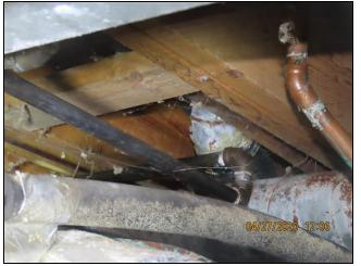
8.1 Item 2(Picture) Corrosion at duct work visible from crawlspace
