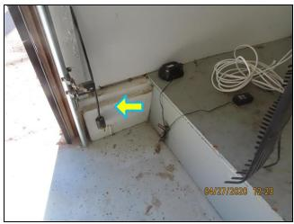
7.0 Item 2(Picture) garage, extension cord may be used at permanent wiring
