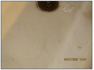
6.2 Item 6(Picture) debris in water supply, upstairs bathroom
