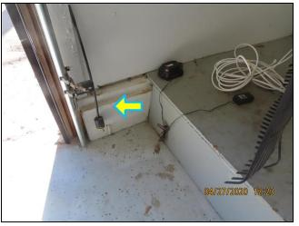
7.0 Item 2(Picture) garage, extension cord may be used at permanent wiring
